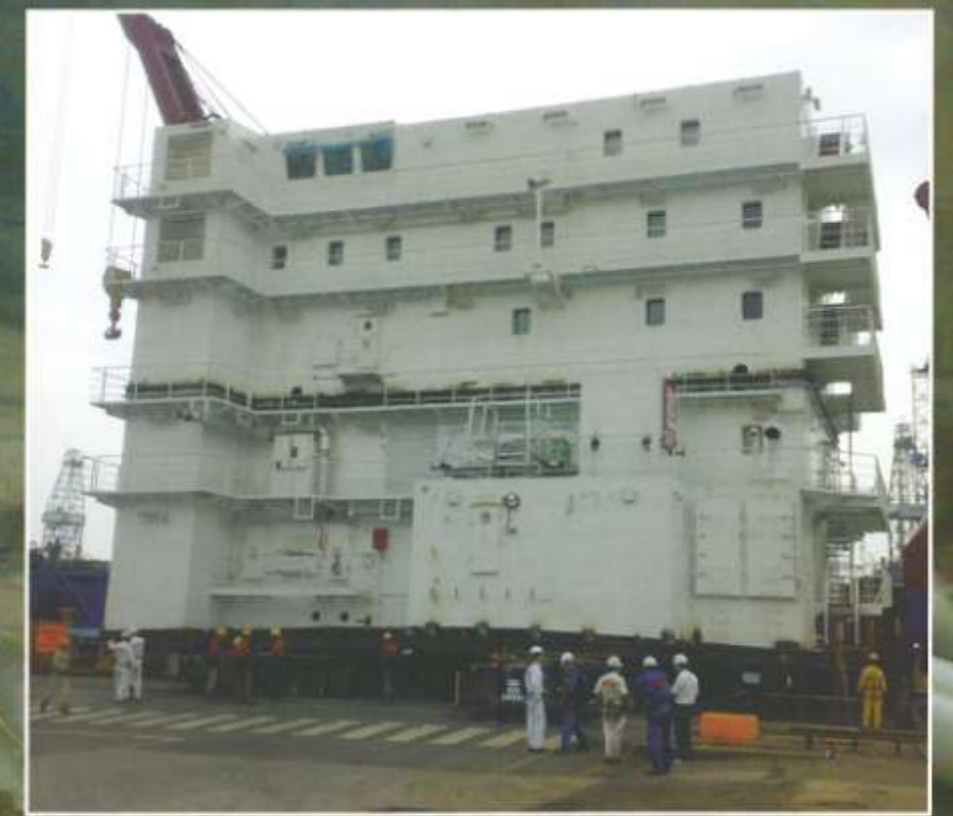
Shifting of Accommodation Block within shipyard (500 Tons).
