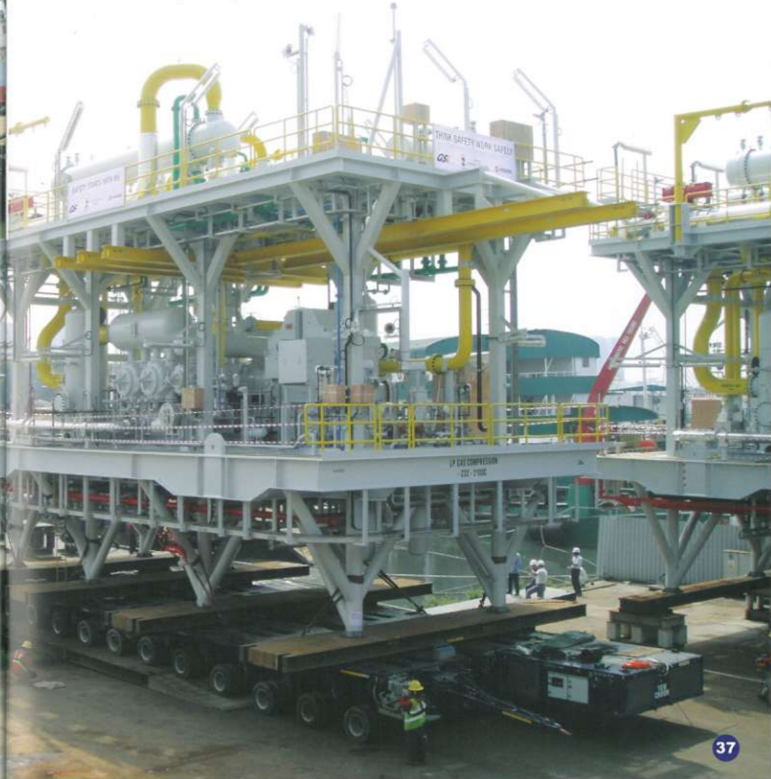
2 units Module being loaded onto barge for sea transportation to Jurong Port. Dim. 17m x 10.5m x 11.5m (300 Tons) each.
