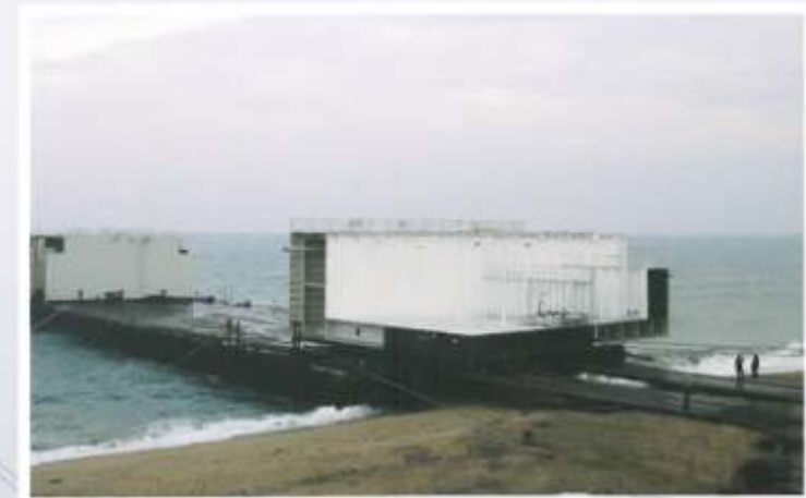
Load-in of second Block. Dim. 22.4m x 21m x 7.78m (218.39 Tons).
