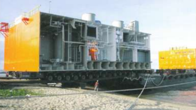
Another successful operation with 2 units Block loaded. Dim. 26.5m x 21.5m x 7.6m (491 Tons) each.
