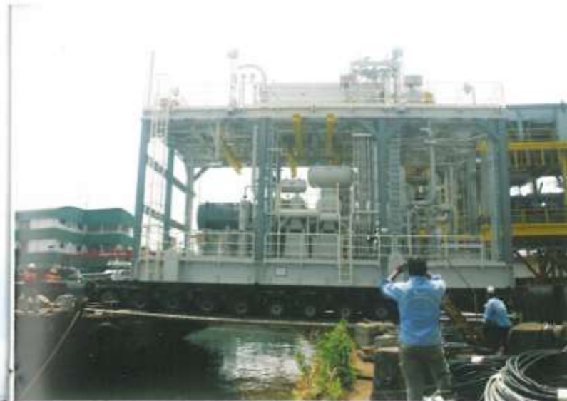
2 units Module being loaded onto barge for sea transportation to Jurong Port. Dim. 17m x 10.5m x 11.5m (300 Tons) each.
