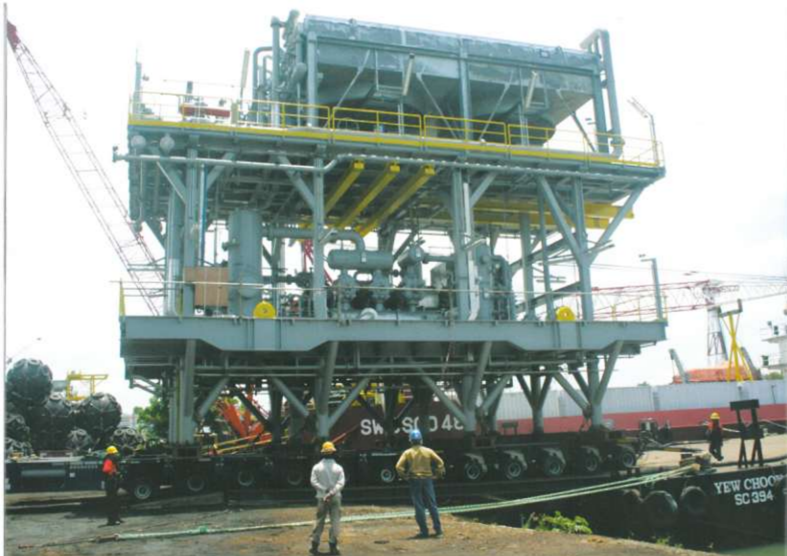
2 units Module being loaded onto barge for sea transportation to Jurong Port. Dim. 17m x 10.5m x 11.5m (300 Tons) each.
