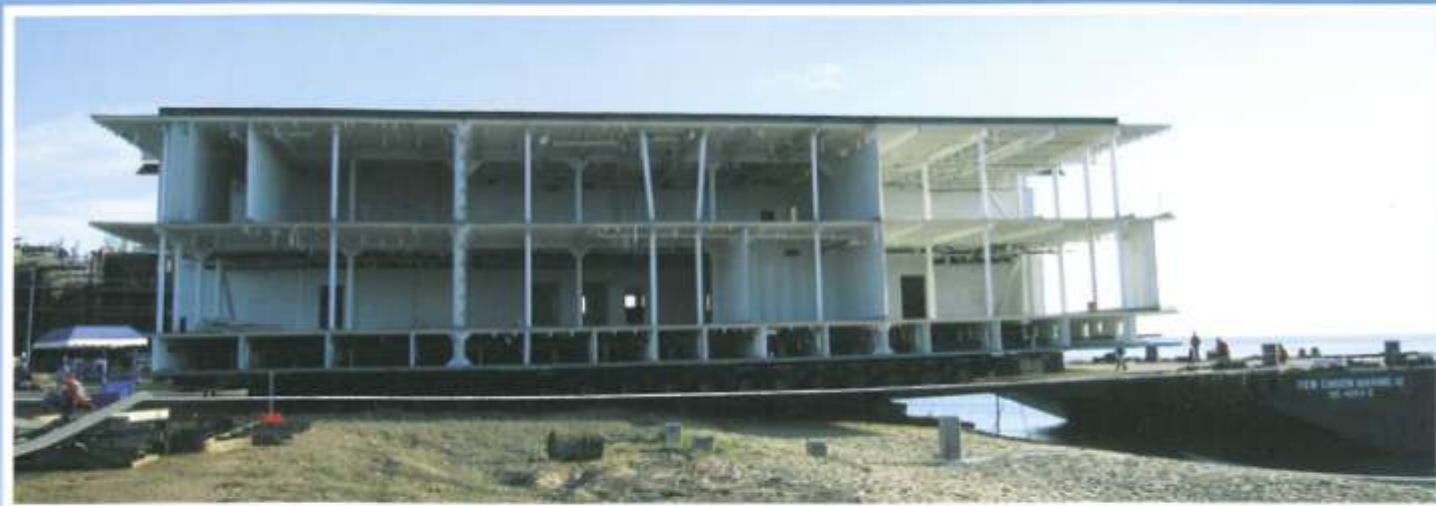
Load-in of cargo onto barge by ro-ro system at temporary landing point. Dim. 35.1m x 14.05m x 7.7m (350 Tons)
