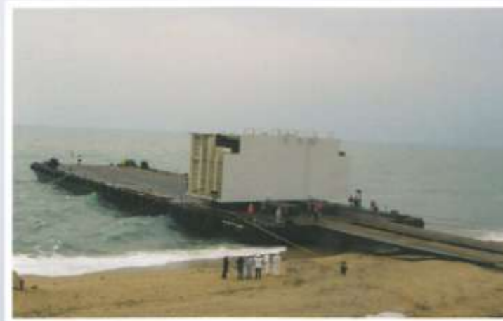
Load-in of first Block. Dim. 8.84m x 20.27m x 7.78m (216.16 Tons).
