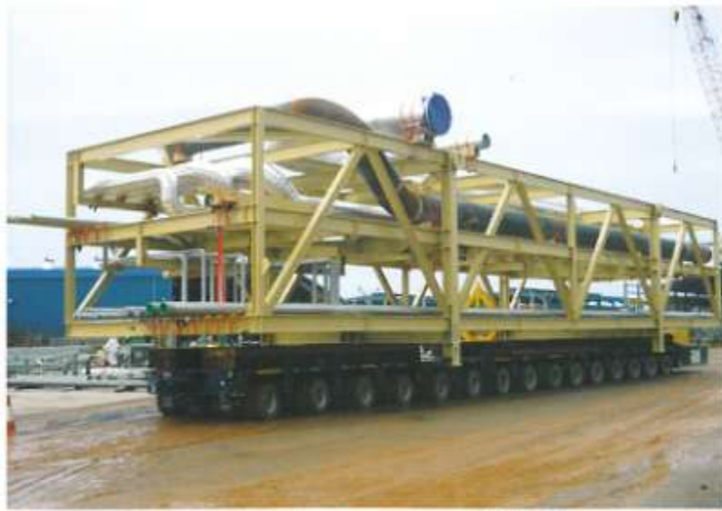
Handling of 145 units PAR Modules, weight from 10 - 280 Tons by 600 Tons crawler crane, 30-axleline PST Goldhofer and barging.
