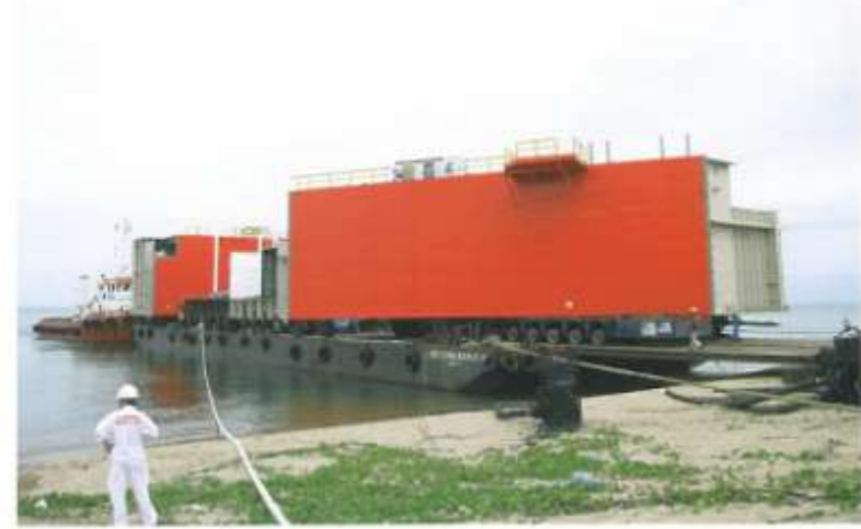
Loading of 3 units Legwell in progress for sea transportation to Singapore. Dim. 8.8m x 20m x 7.7m (160 Tons), 19.6m x 21.5m x 7.7m (220 Tons) and 19.6m x 21.5m x 7.7m (220 Tons).
