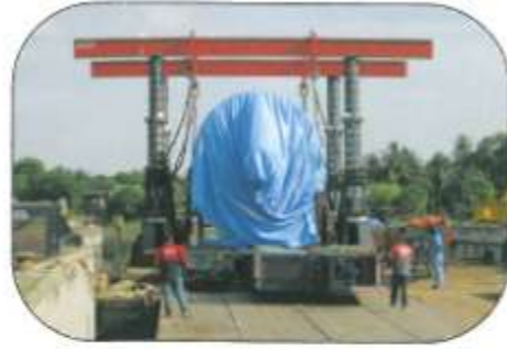
Lifting turbine on trailer.
