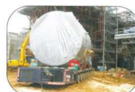
Delivery to site.
