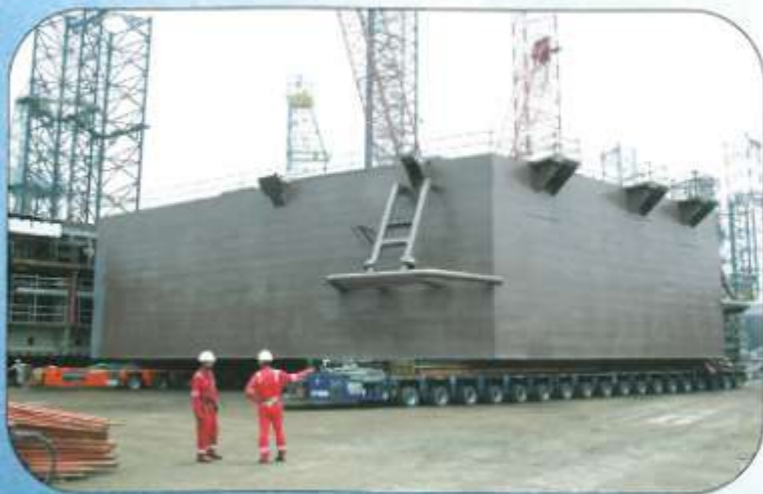
Singapore PPL Shipyard assigned Yew Choon to shift this 700 tons Legwell within the yard.
