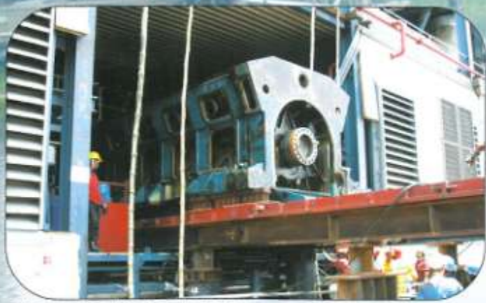
Old engine block skid-out.
