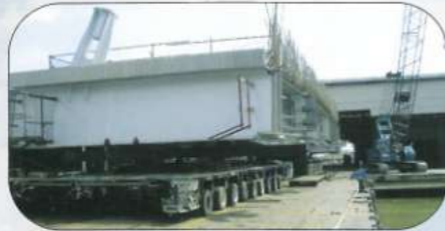
At the jetty, load-in of cargo onto barge.
