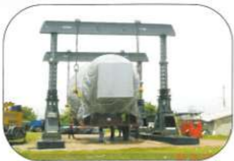
Jacking by 600 tons 4-point lift system...
