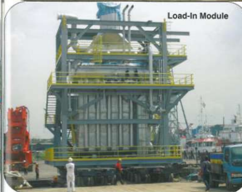
Site move by 2 self-propelled hydraulic trailers
