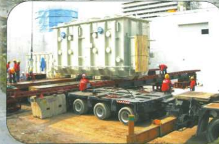
Transformer skidded to position.
