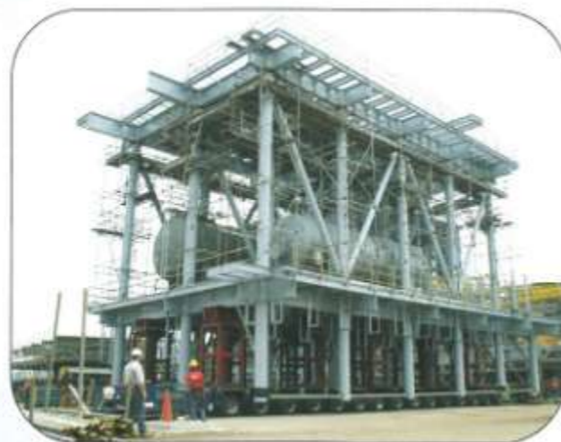
Singapore Yew Choon moved 14 units of these Modules and Structures from the storage area to the sea-front. The biggest is 850 tons, 29.5 x 19.3 x 12m.
