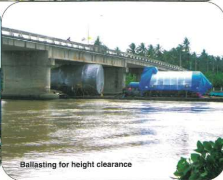
After assembly, load-on to barge for transport to site
