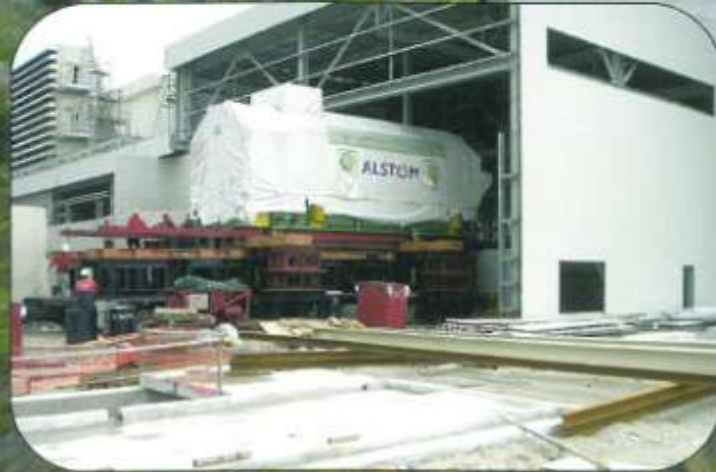
Position of 320 Tons Generator onto foundation by skidding system.
