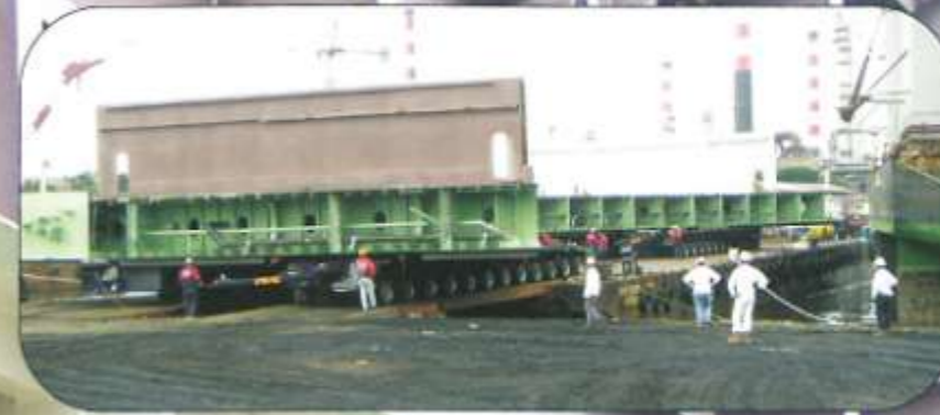
Singapore One of 5 Heavylifts, total weight: 1,126 tons delivered to PPL Shipyard from UDI Shipyard.
