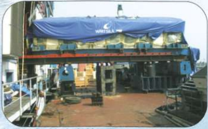
New engine block skid-in.
