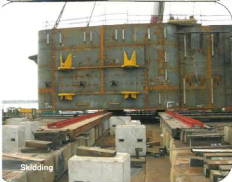
After assembly, load-on to barge for transport to site
