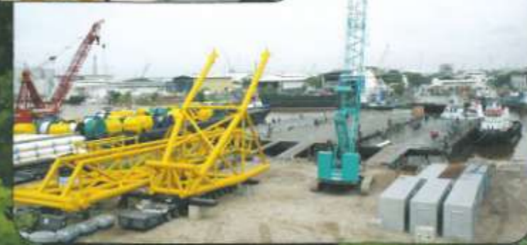
Barge, tug boat, hydraulic trailer and crane
