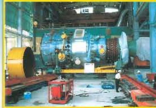
Moving 375 tons Gas Turbine into position by hydraulic pushing jacks on skids.
