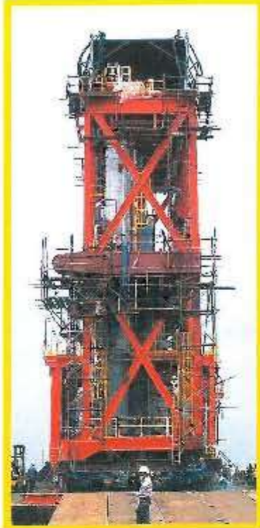
Re-ro ramps in place for this 590 tons Module. Dimension: 16 x 7 x 26m.
