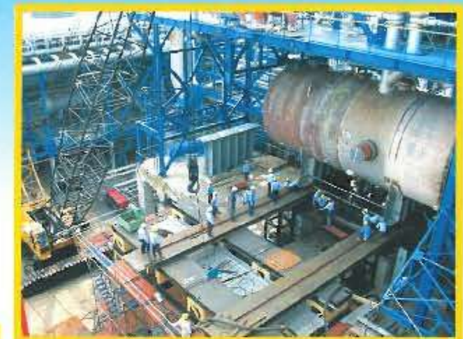
Yew Choon constructed a 10m high platform next to the foundation of the old heat exchanger.
