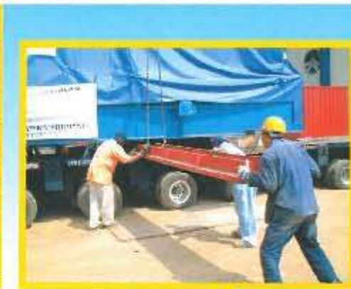
Positioning of the skidding channel.
