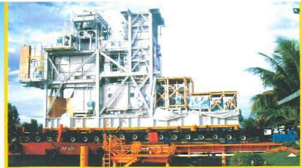
Ro-ro operation of Turbo Compressors on arrival in Senpah.
