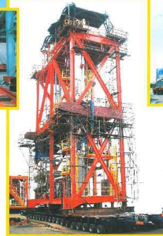
Moving 375 tons Gas Turbine into position by hydraulic pushing jacks on skids.
