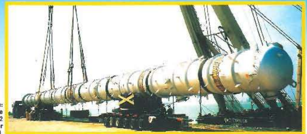
Transporting this 319 tons Unit to site by self-propelled trailer (spt) with heavy duty turntables.
