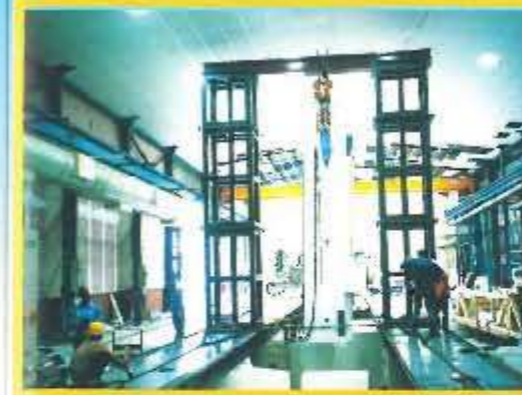
Positioning in progress.
