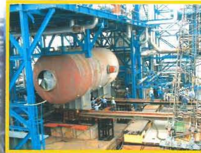
The old heat exchanger was skidded onto the platform...
