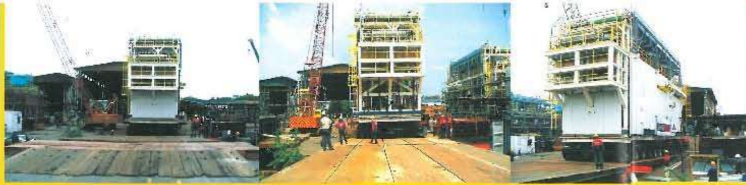
Roll-on of 289 tons Gas Compressor to barge for journey to Hazira, India. Dimension: 25 x 7.8 x 11.7m.
